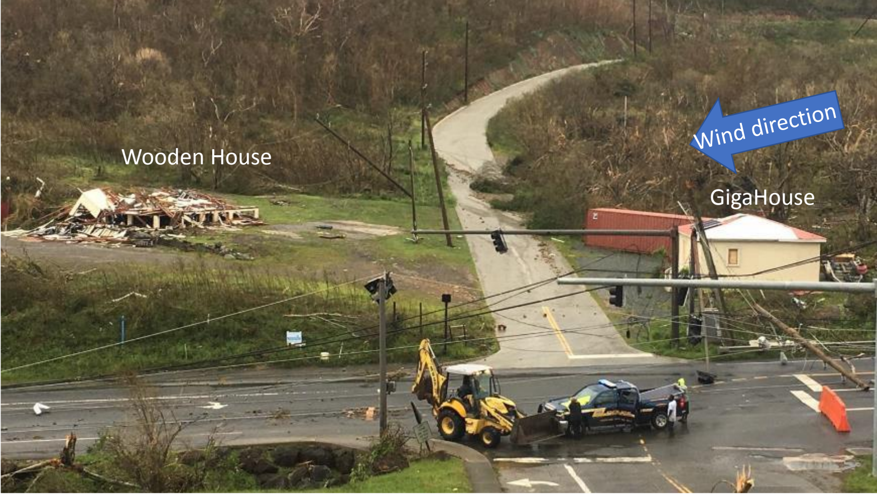
St Thomas USVI GigaCrete Caribbean Sales Office after Hurricane Irma and Maria, note the stripped trees everywhere and the wood framed building across the street, completely destroyed.
